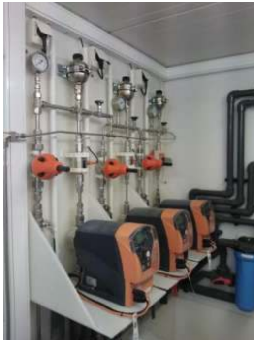
Feeding equipment installed in a container for three different feeding locations in one system
